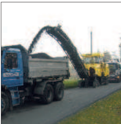
Milling, sweeping and paving in quick succession.
