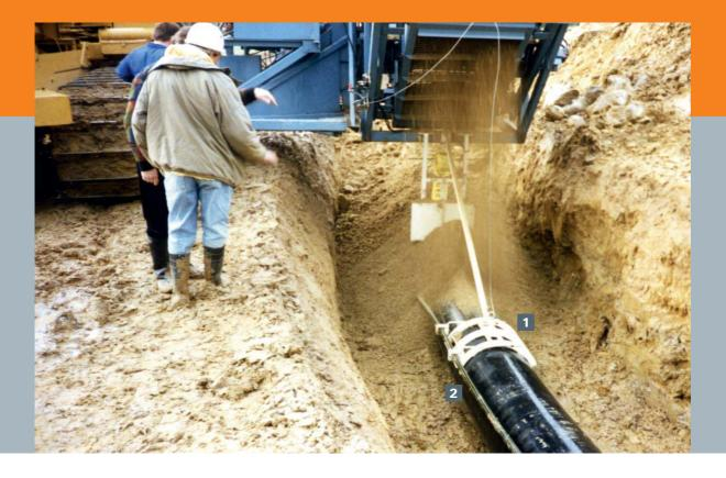
KNI dynapad integrates the laying of geotextile fabric, of glass fiber conduit and of warning tapes. KNI dynapad's patented collapsible pipe supports give additional advantages for bedding and natural compaction.
