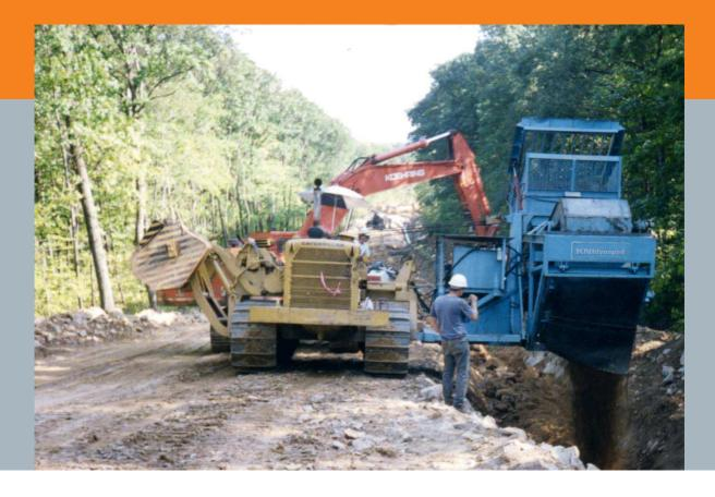
The KNI dynapad technology for bedding, padding and backfilling gives premium advantages to reduce costs and enhance the quality and safety of pipeline construction and operation with its layered filling principle. The modular construction allows the usage of KNI dynapd's unique collapsible pipe supports and the integration of geotextile fabric and cable laying.
